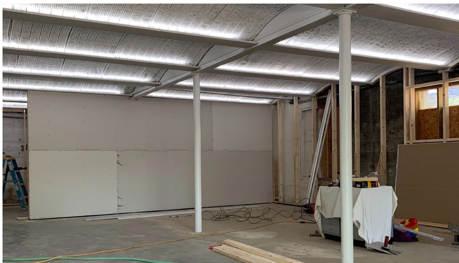
Alexander Gray Associates, Germantown under construction (2020)
